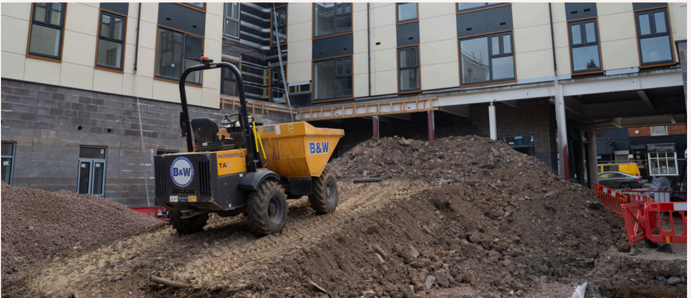
Construction at SCD, 2025
