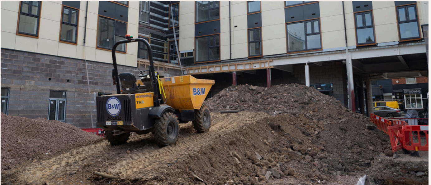
Construction at SCD, 2025
